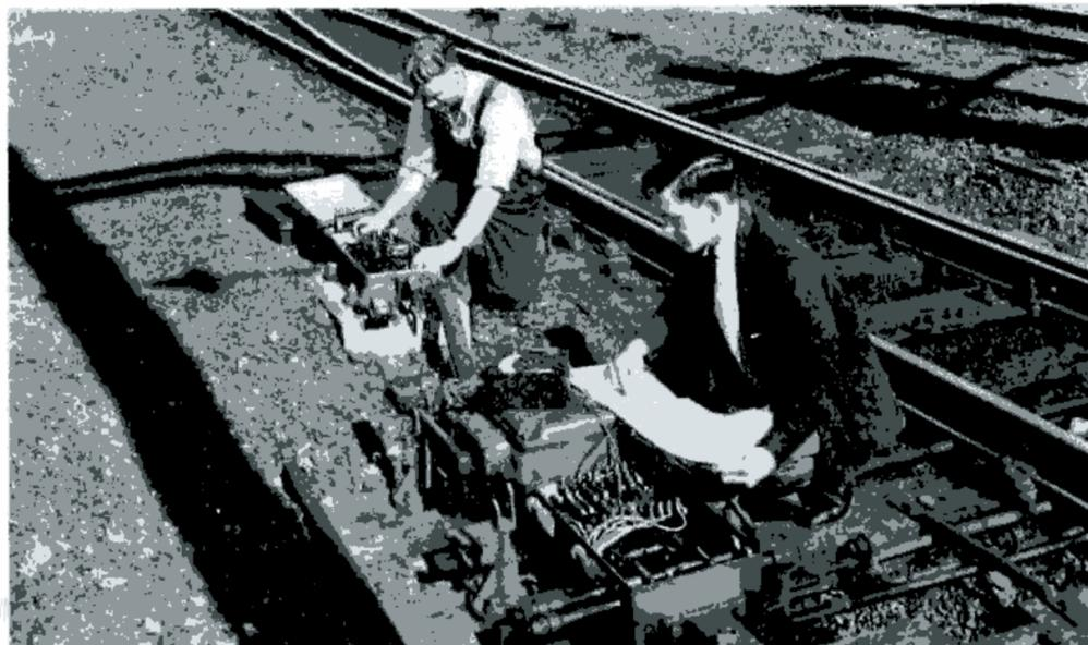
Railway signal engineering is interesting and diversified. Here an engineer and a signals maintainer test and adjust an electric points motor.
